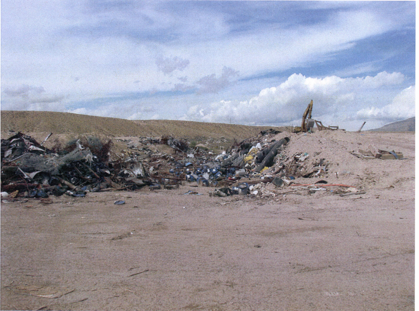
Looking west at the working face. The backhoe was placing cover soil during the site visit.
